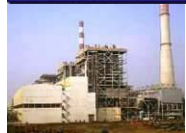
Zouxian Power Plant Largest pulverized coal-fired utility boilers in China
